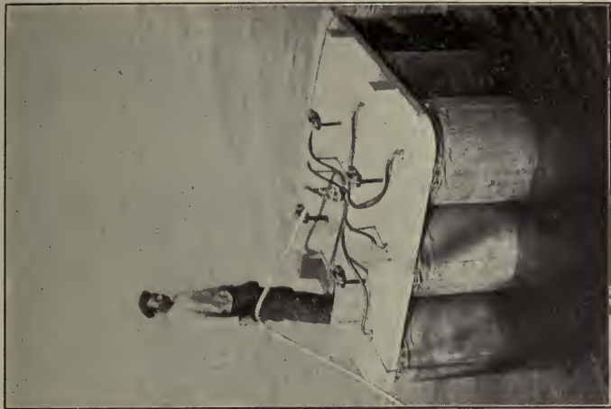
An "elevator" with air bags inflated. Photographed in Vigo Bay.
